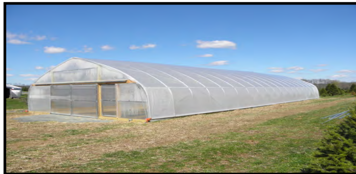
This Season High Tunnel was the first installed in NJ in Cream Ridge
