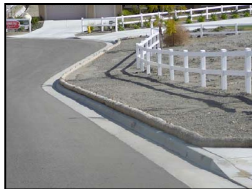
Sediment barriers, like the wattle bordering the curb above, may be tested at Rutgers University.
