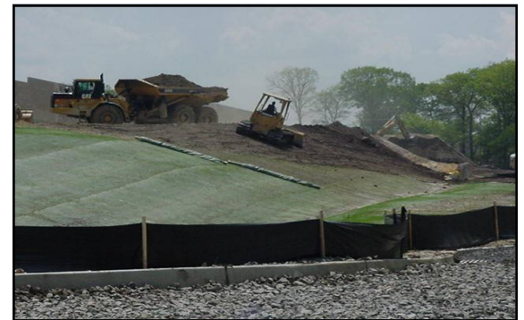
Erosion controls in place
