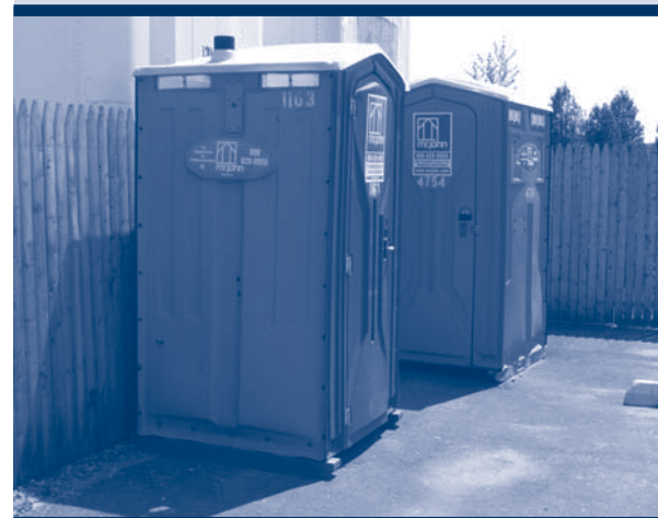
Properly Located Restroom Facilities on a Solid Surface
