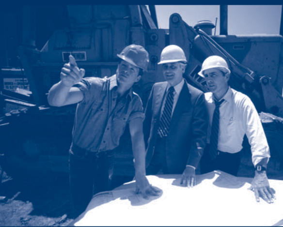
Weekly Inspections by the Builder's On-site Representative are Needed to Manage and Control Stormwater Pollution
