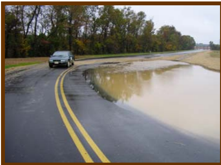
Sediment and water runoff from a construction site onto a roadway can cause hazardous conditions for motorists.
