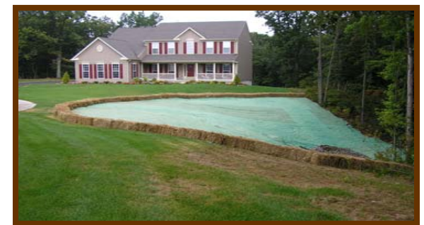
The use of erosion matting for slope protection provides successful erosion control and prevention of sedimentation to the adjoining woodland.
